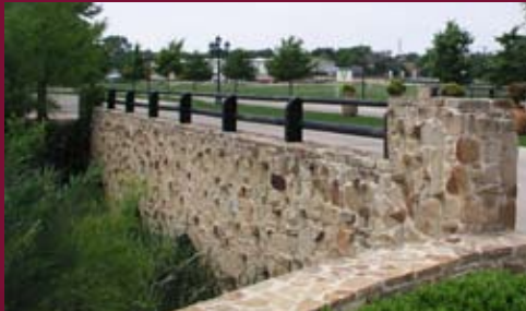
Colleyville Church St. Roadway Reconstruction and Mission Lane Bridges – Civil engineering design services for roadway reconstruction which included two bridges and realignment of an older segment of Church Street with a newer portion of the roadway by developing a tight reverse curve design with super elevation.
