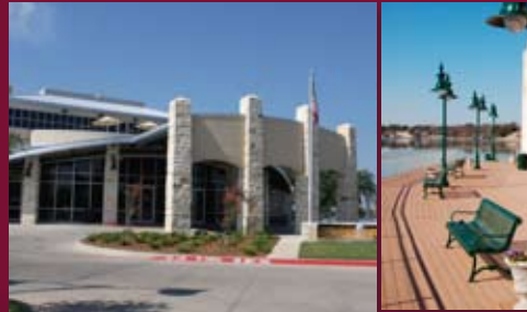
Granbury Resort Conference Center and Boardwalk – Survey, Civil and MEP engineering design services for the 15,000 SF, two-story conference center and boardwalk located on the shores of Lake Granbury in historic Granbury. This project redeveloped an older, poorly utilized site into a new, upscale amenity for Granbury.
