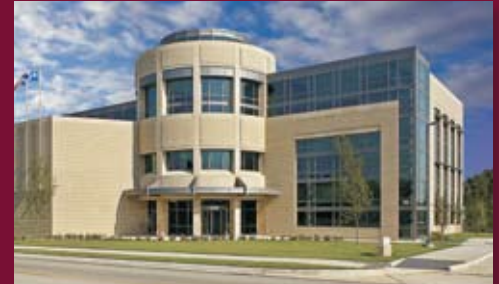
Tarrant County SE Sub-Courthouse - MEP and security systems engineering design services for a new, $10 million, 50,000 SF Sub-Courthouse which received LEED Silver Certification and is the first building in Arlington, for Tarrant County and the first Courthouse in Texas to be LEED Certified. (Annual energy consumption reduced by 38.6%, resulting in an annual cost savings to the Owner of 21.8% on energy bills)
