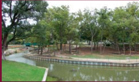
Granbury Riverwalk Hike & Bike Trail - Survey and Civil engineering design of a 10' wide concrete hike and bike trail along Lambert Branch which included a crossing under the existing bridge on FM 51. At the time of the excavation, a historic limestone retaining wall was discovered requiring a rapid redesign of the soil nail wall to preserve this historic element.
