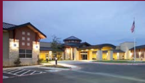
North Texas Medical Center , Gainesville, TX - Site/Civil and MEP engineering design for this 115,000 SF, $16 M replacement Hospital Design included HVAC, medical gases, fire sprinkler, domestic water, sanitary sewer, hot water, lighting, power, fire detection and alarm, nurse call system, code blue and paging. Emergency power systems consisting of a diesel drive emergency generator, three automatic transfer switches and one manual transfer switch were also included.
