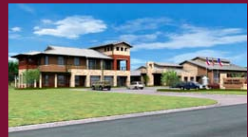
Grand Prairie Fire Rescue Station , Grand Prairie, TX - Site/Civil and MEP engineering design for the new $6 M, 20,780 SF facility designed to achieve LEED Silver Certification to house a fire station, a police department, a lake parks admin. building and a lake parks service bay building on approximately 4.3 acres. Geothermal heat pumps were used and are predicted to reduce annual energy consumption by 19%, reduce water usage by 35%, and increase ventilation rates by 30%.
