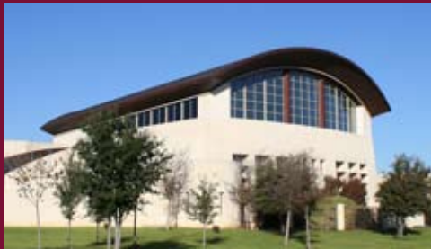
Beth-El Congregation , Fort Worth, TX - MEP engineering design for this 45,000 SF facility. Many specialized designs were utilized for this project such as the building of a concrete tunnel for a return air path from the sanctuary. This was done instead of using fiberglass ductwork in order to save on construction cost. BHB's team designed in accordance with the sensitive acoustical requirements for several areas of the building.
